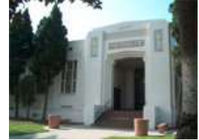
Franklin Elementary School in Santa Ana, California.
